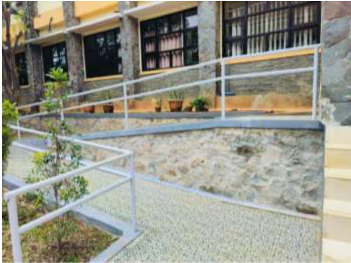
Gambar..... Ramp Disabilitas Gedung TIP
